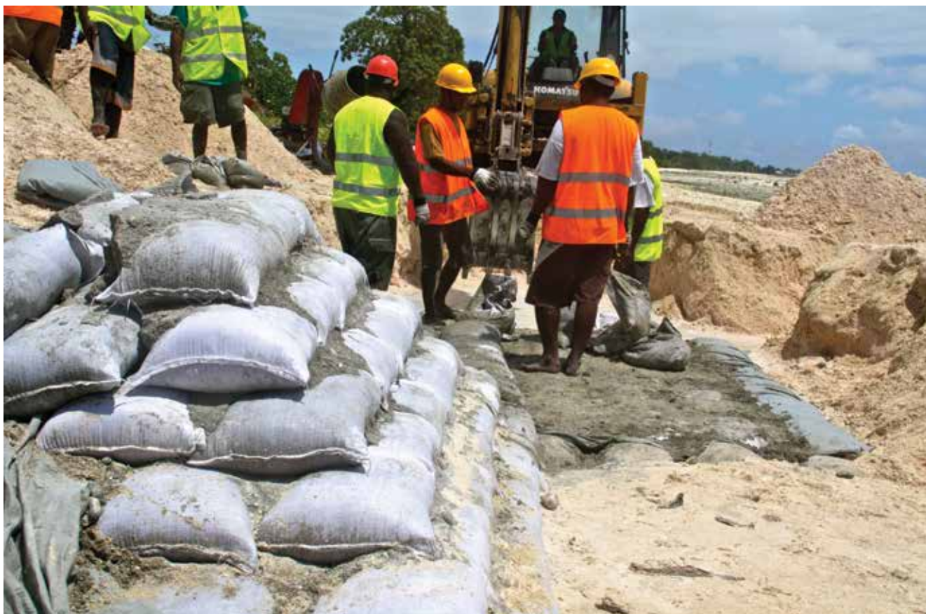
Building Seawalls. Tarawa, Kiribati.
